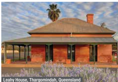
Leahy House, Thargomindah, Queensland
